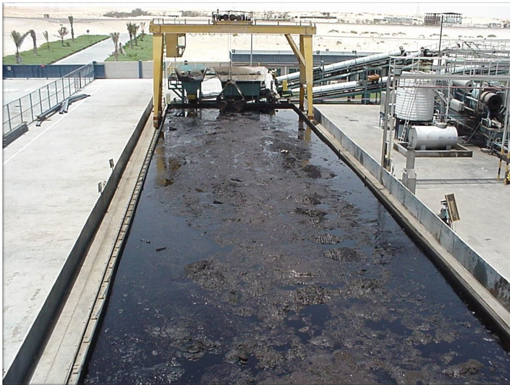
Drill cuttings in receiving pit prior to treatment
